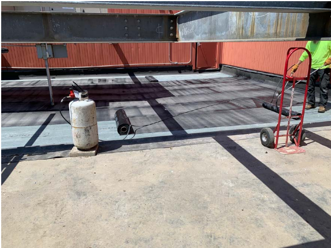
Recreation Center Roof Replacement
