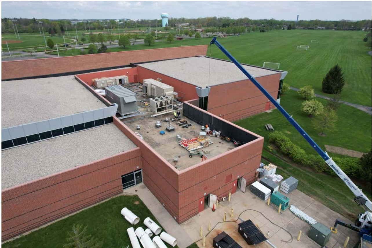
Recreation Center Equipment Installation
