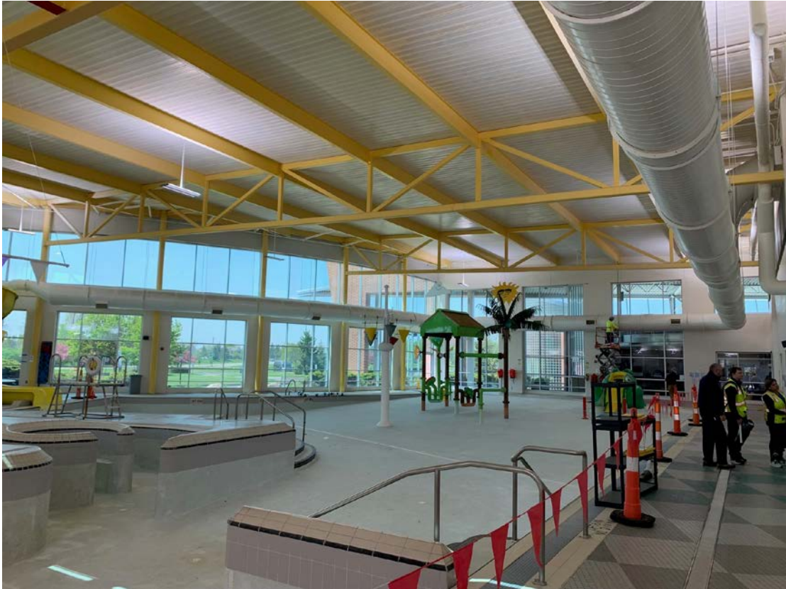
Pool Duct Removal
