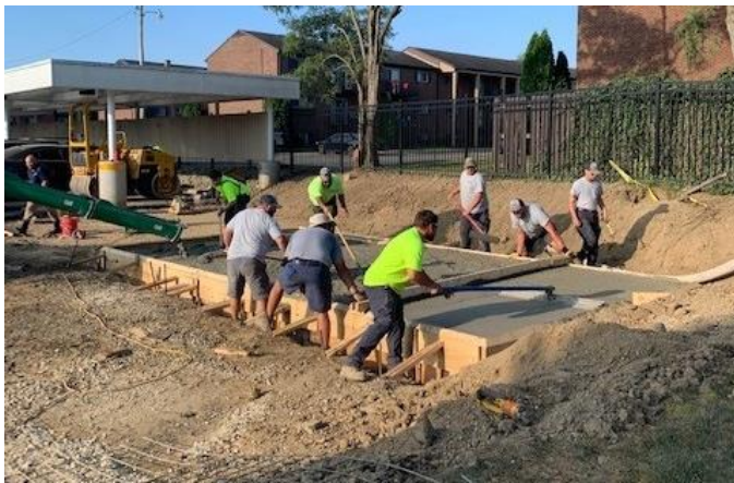
Parks & Recreation and Public Works staff working to complete the concrete pour for the Police Department Shed at the Justice Center. Teamwork makes the Dream Work.
