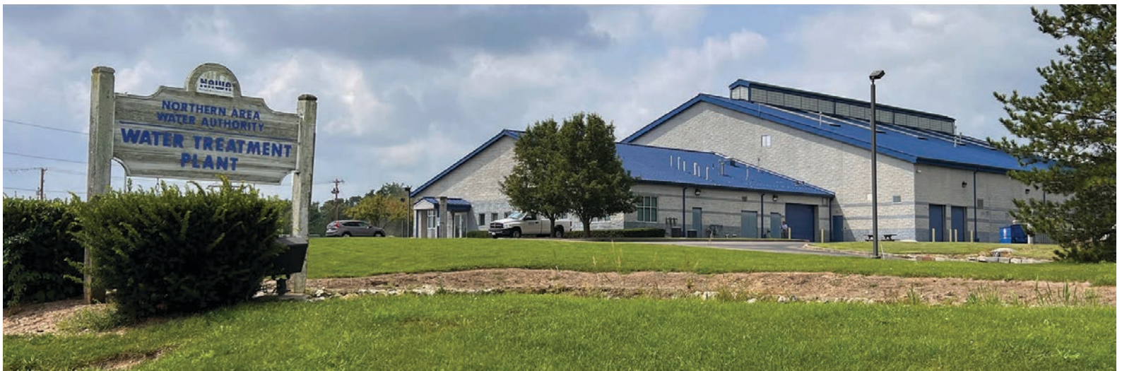
The Northern Area Water Authority (NAWA) Water Treatment Plant, a joint project between Vandalia and Tipp City, is located on Canal Road in Tipp City.
