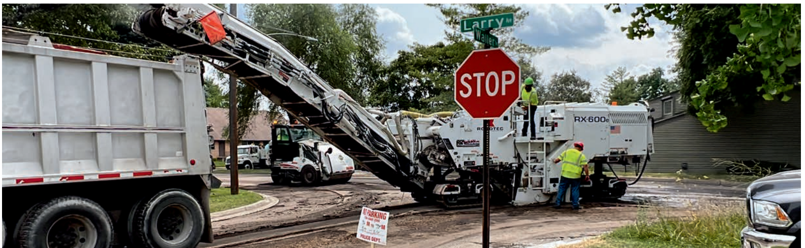
Vandalia utilizes Safe and Stable funds to resurface a number of City streets each year.
