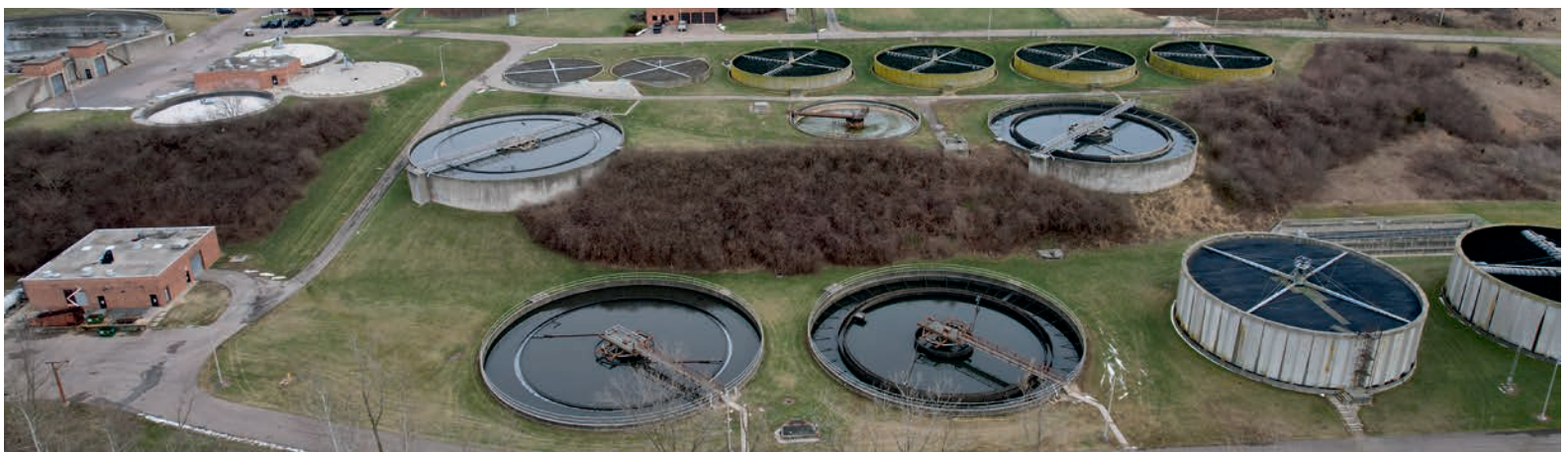
The Tri-Cities Wastewater Treatment Plant is jointly operated by the cities of Vandalia, Huber Heights and Tipp City.
