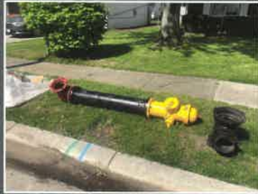
(Above) New fire hydrants were installed as part of a water main replacement project on Marview Avenue.
