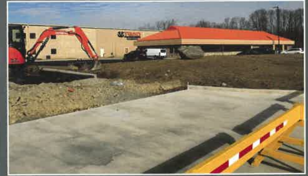
(Above) Triad Technologies is in the process of completing a 47,000 sq. foot expansion in 2020, which nearly doubles the size of its Vandalia operation.
