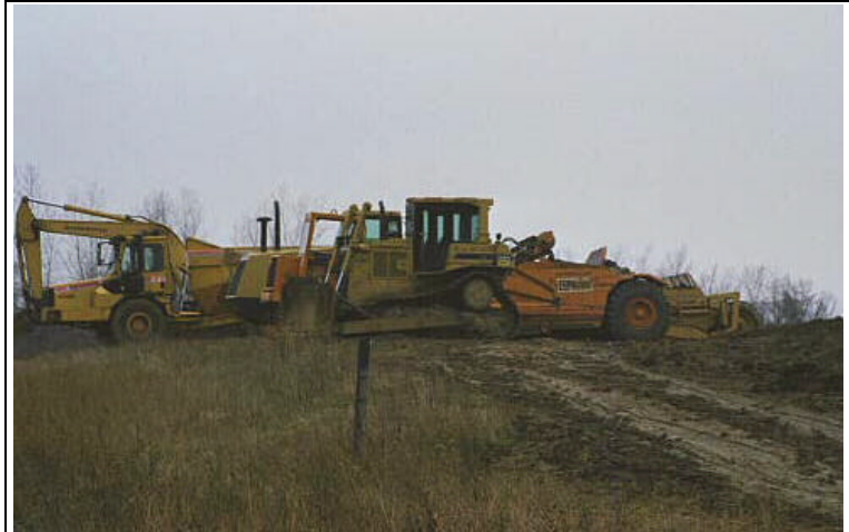
Area under construction off Brown School Road.
