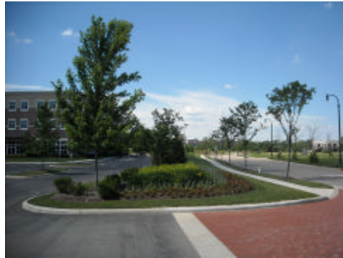
Figure 7: Brick pavers used to emphasize major intersections and crosswalks.
