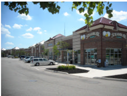
Figure 15: Retail building with roof height and elements. roof pitch variations.
